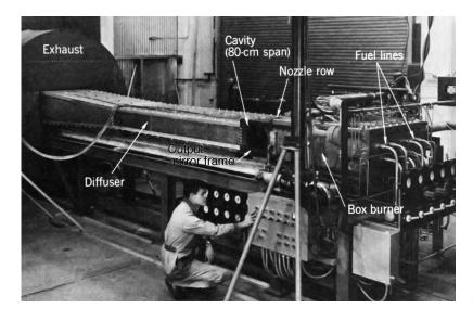
Fig. 7. An experimental gas-dynamic CO<sub>2</sub> laser developed by AVCO Corporation circa 1968. The output was over 50 kW.
